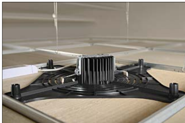
SpotClip-Plate til tunge downlights.
